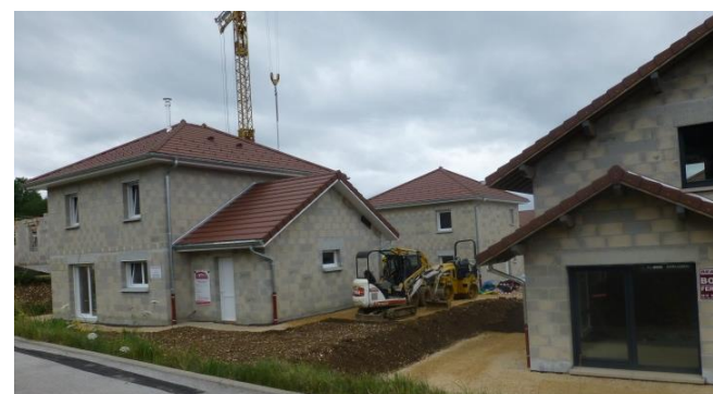
Construction neuve, Granges-Narboz
